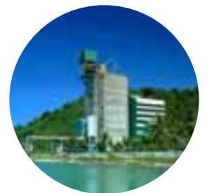
Terminal Lembar, Lombok Lembar Terminal, Lombok
